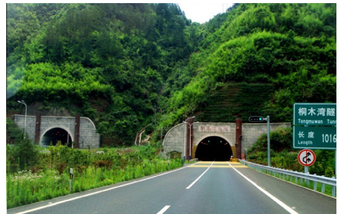
Fig. 26. Portal of Tongmuwan tunnel ( http://tcliuke.blog.163.com/blog/static/677638672010101483328691/ ).
