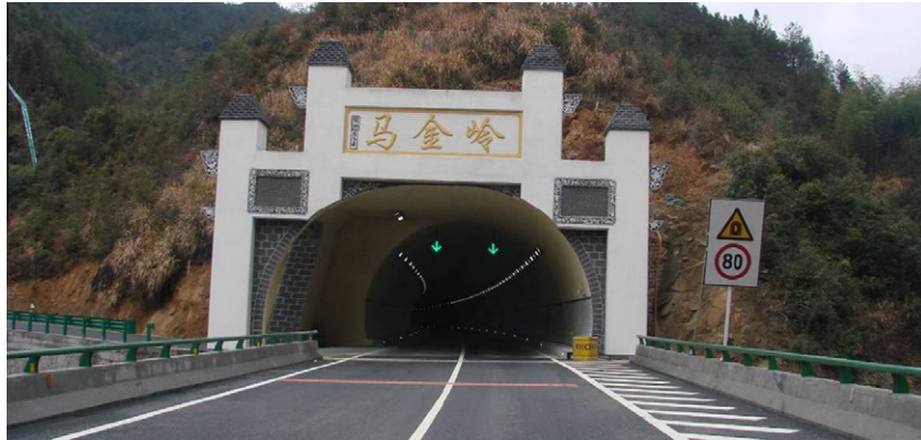
Fig. 21. Portal of Majinling tunnel (Liu et al., 2010).
