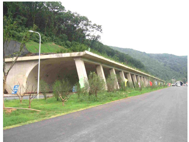
Fig. 32. Photo of Laoshan No. 2 tunnel.
