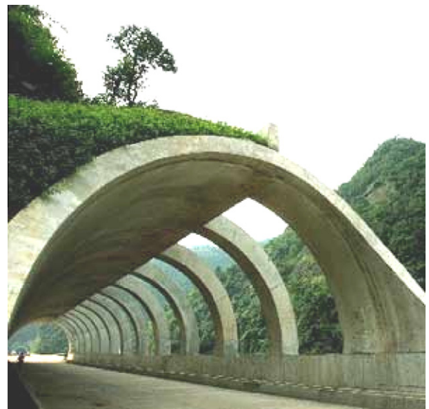
Fig. 33. Photo of Longpu tunnel.
