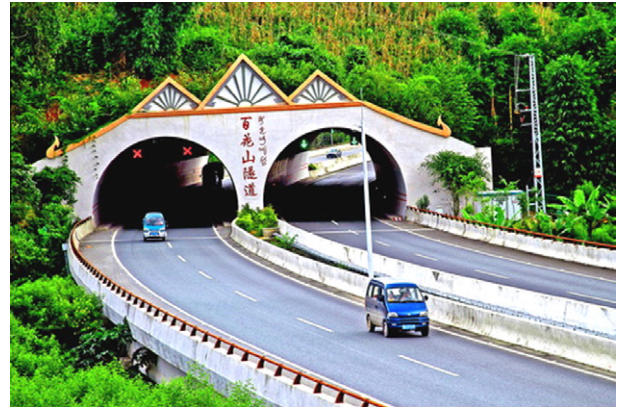
Fig. 10. Portal of Baihuashan tunnel with Dai nationality architectural factors ( http://lvyou.wanjingchina.com/bencandy.php?fid=40&aid=136530&page=3 ).
