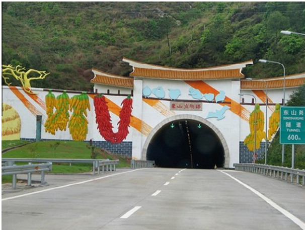
Fig. 24. Portal of Dongshangang tunnel (the image was provided by Zhang, L. C.).
