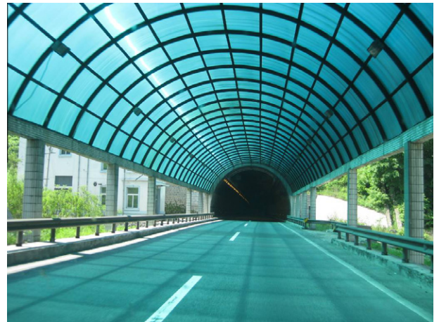
Fig. 35. A shading structure between tunnel portals in a tunnel group.
