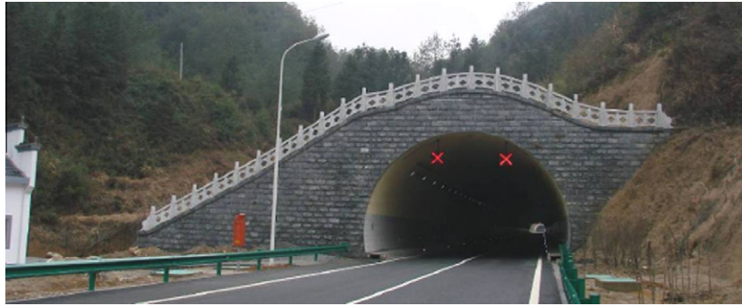
Fig. 18. Portal of No. 1 Guanpujie tunnel (Liu et al., 2010).
