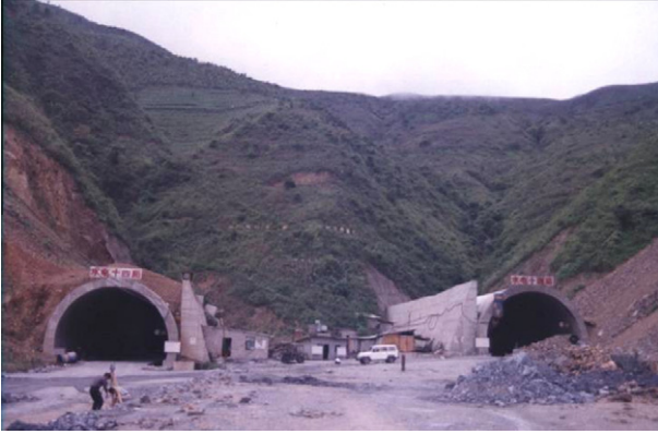
Fig. 2. The highway tunnel portal located in mountain valley.
