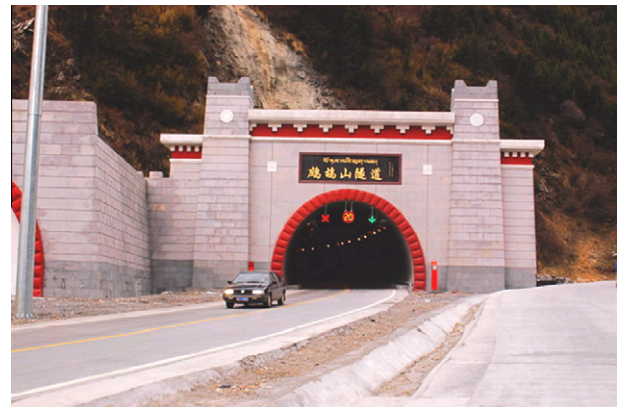
Fig. 17. Portal of Zhegushan Mountain Tunnel (the image was provided by Qiu, Y. L.).
