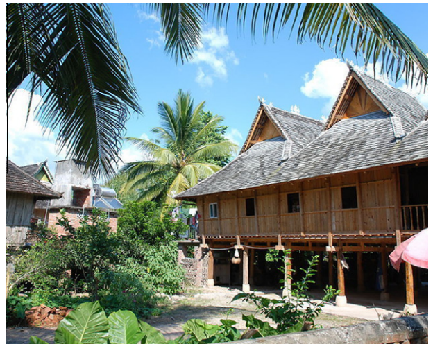
Fig. 11. Bamboo houses of Dai nationality (the image was provided by Zhang, T. Z.).
