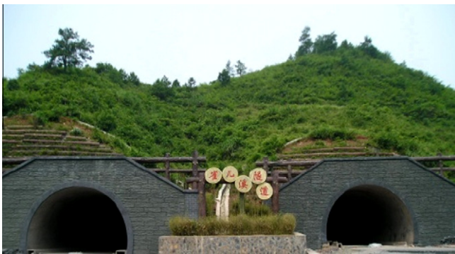
Fig. 25. Portal of Queerxi tunnel ( http://tcliuke.blog.163.com/blog/static/677638672010101483328691/ ).
