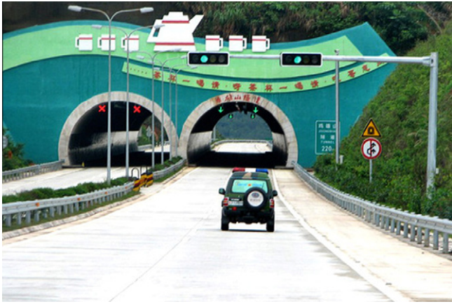
Fig. 28. Portal of Jixiongshan tunnel (the image was provided by Zhang, L. C.).
