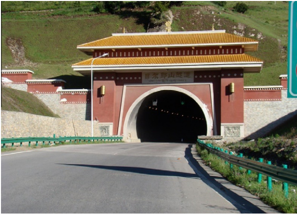
Fig. 13. Portal of Rierlang Mountain Tunnel with typical Tibetan feature ( http://attachments.motorfans.com.cn/2010/10/26/MFMDOV8zt5549.jpg ).
