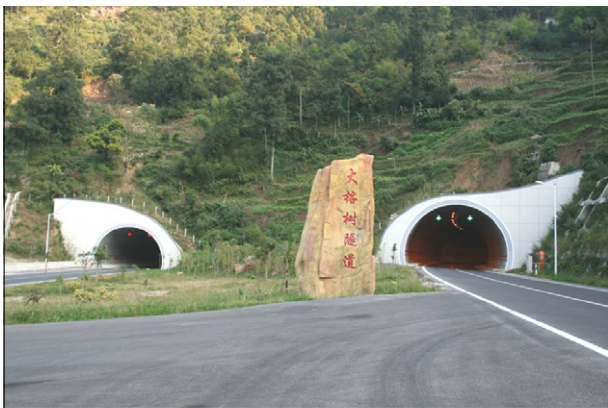
Fig. 8. Linear geometry of tunnel portal (the image was provided by Zhang, T. Z.).
