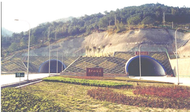
Fig. 6. The naked shotcrete covering slope of tunnel portal.
