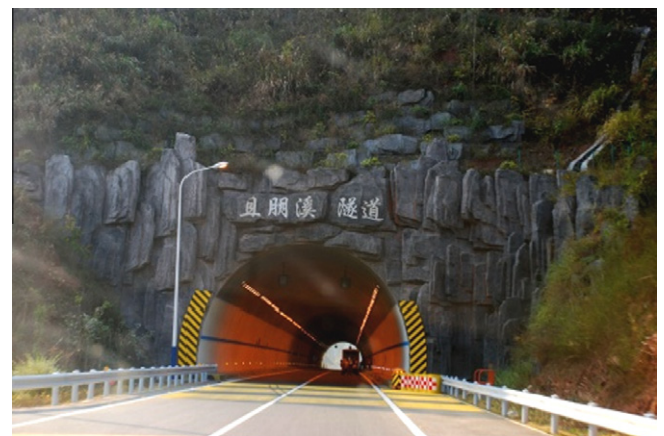
Fig. 37. Portal of Qiepengxi tunnel.
