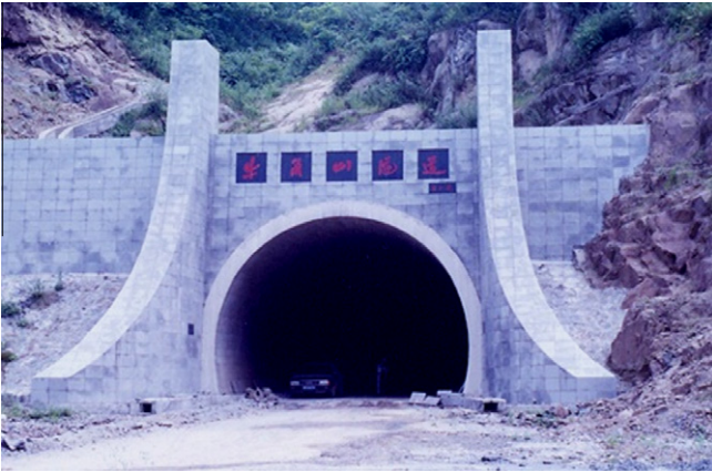
Fig. 39. Portal landscape of the Niujiashan tunnel ( http://www.hczjgs.cn/hczj/T_ProductShow.asp?ProductID=22&SmallClassID=11&BigClassID=44 ).
