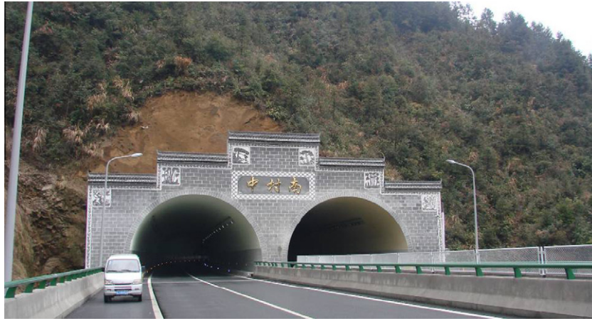
Fig. 23. Portal of Zhongcun tunnel (Liu et al., 2010).
