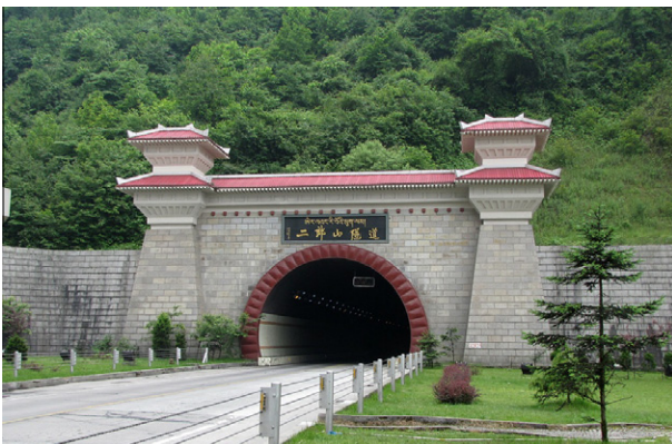
Fig. 15. Portal of Erlangshan Mountain Tunnel ( http://fengyunbike.com/thread-11982-5-1.html ).
